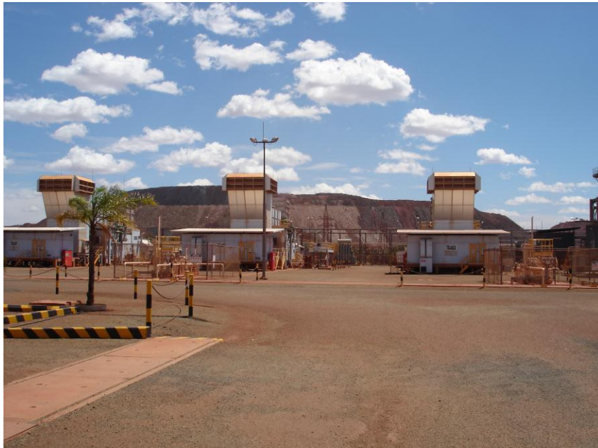
Figure 3: Newman Power Station
