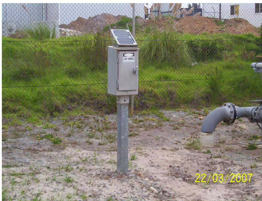
Typical pressure monitoring installation
