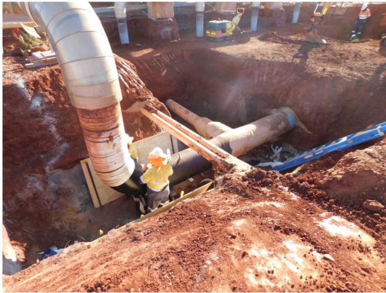
Unit discharge pipework exposed to access areas with high gas temperatures
