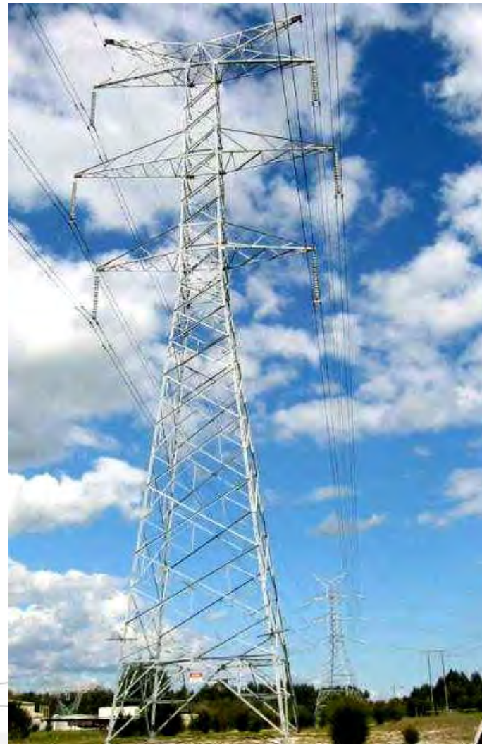
A 330kV structure
