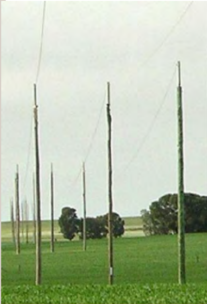
132kV existing line
