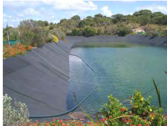
Image 2. Northern water reservoir showing neoprene lining and lowered water supply.
