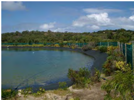
Image 1. Southern water reservoir. The clubhouse roof is visible at right on the horizon.
