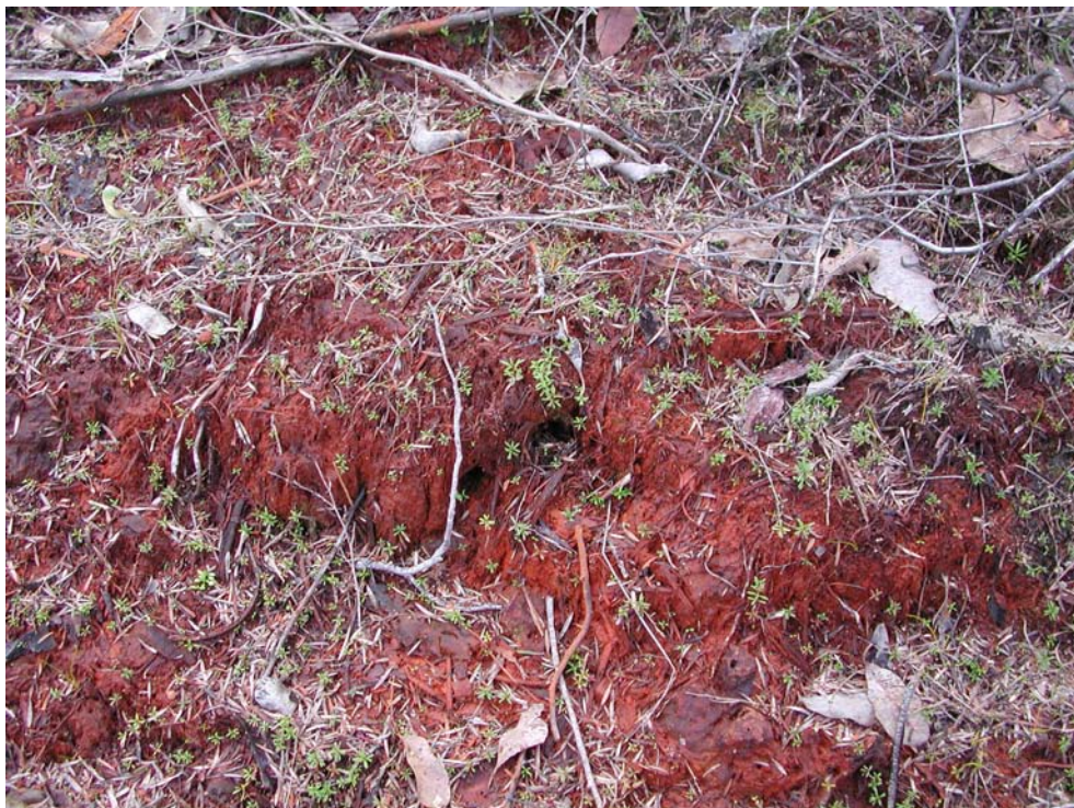
Plate 4.2: Seepage holes within the right abutment downstream of the embankment
