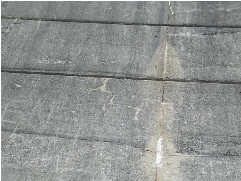
Plate 4.11 Minor AAR Cracking on Downstream Face
