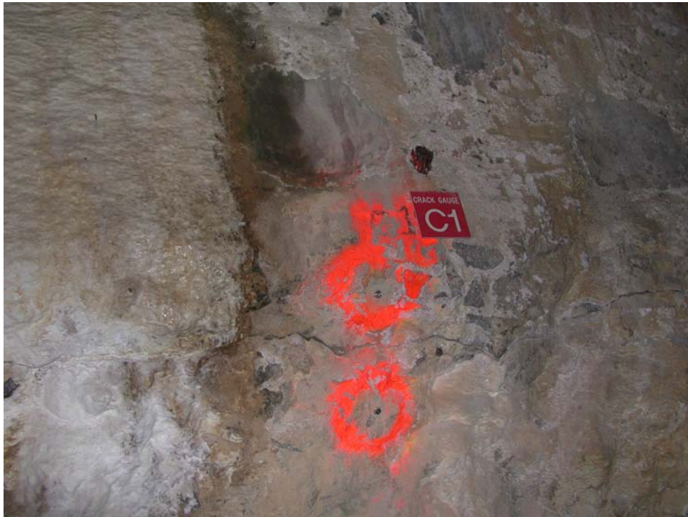
Plate 4.10 Cracking at base of original dam
