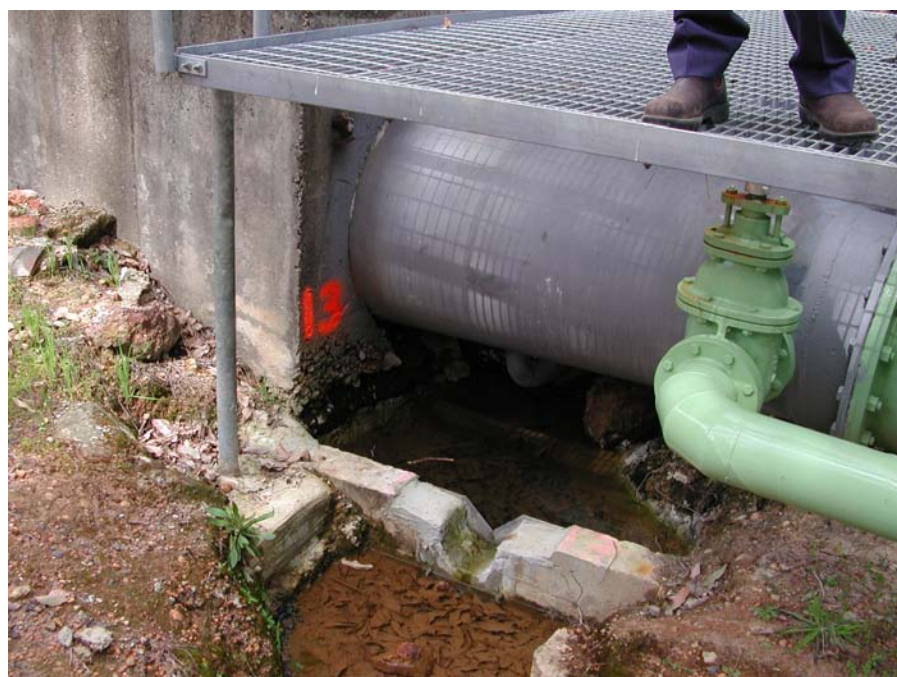
Plate 4.14 : Minor Seepage Along Conduit at Samson Brook
