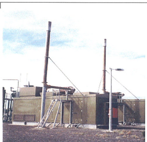
600 kW generating plant fuelled by biogas
