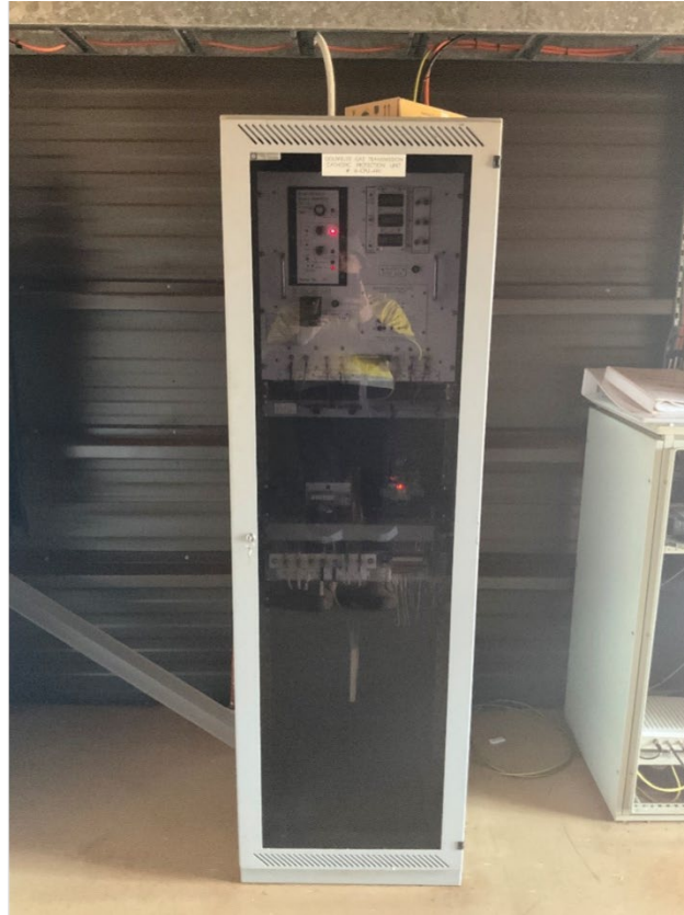
Figure 2 CP Unit at Newman Scrapper Station
