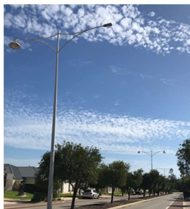
Figure 1: Example showing a luminaire installed by the land developer initially and then replaced by Western Power with two different types of luminaires over time.
