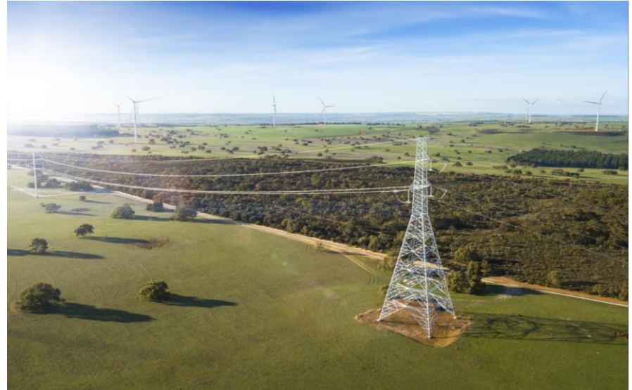
Transmission towers (Yandin windfarm)
