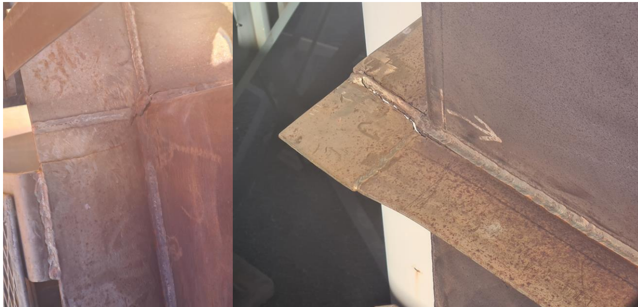
Figure 2: Sectional flange cracking on CS3 U1 (August 2020)
