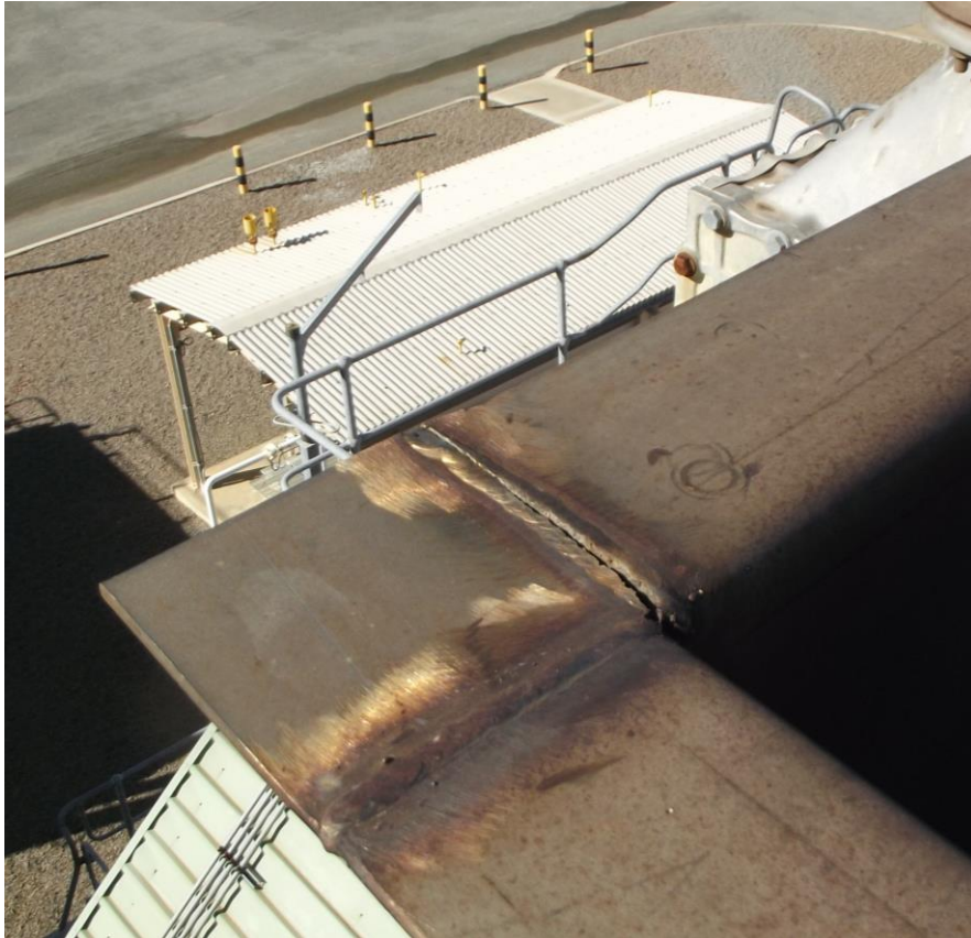
Figure 7: Top flange cracking CS8 Unit 1 (2020)
