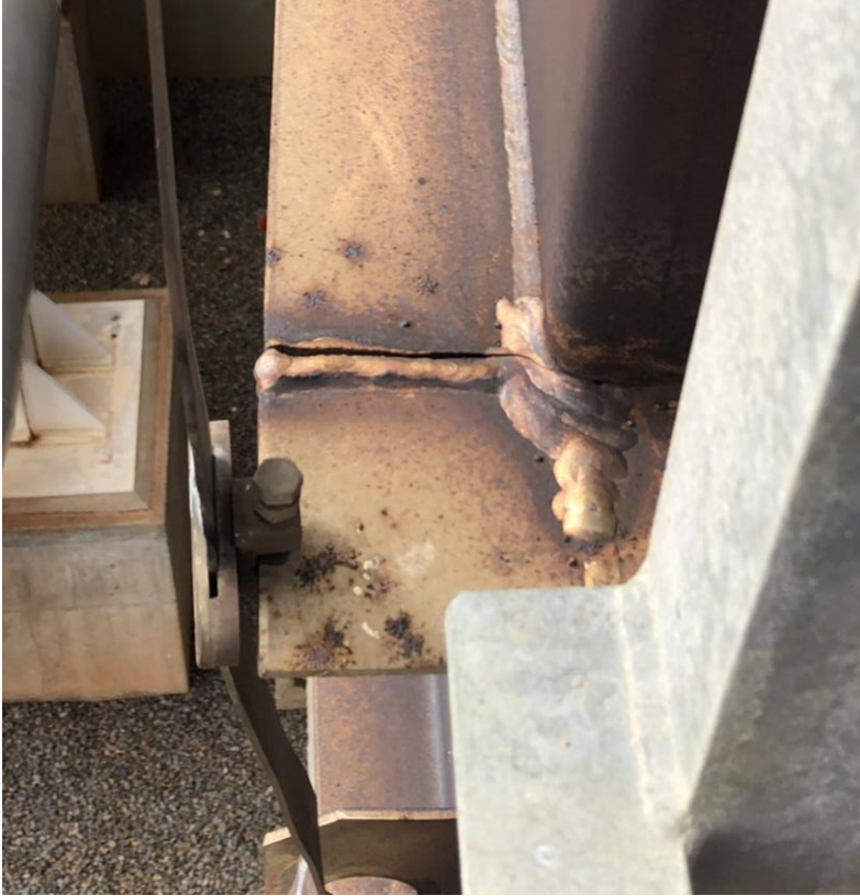
Figure 5: Sectional flange cracking CS5 Unit 2 (August 2019)
