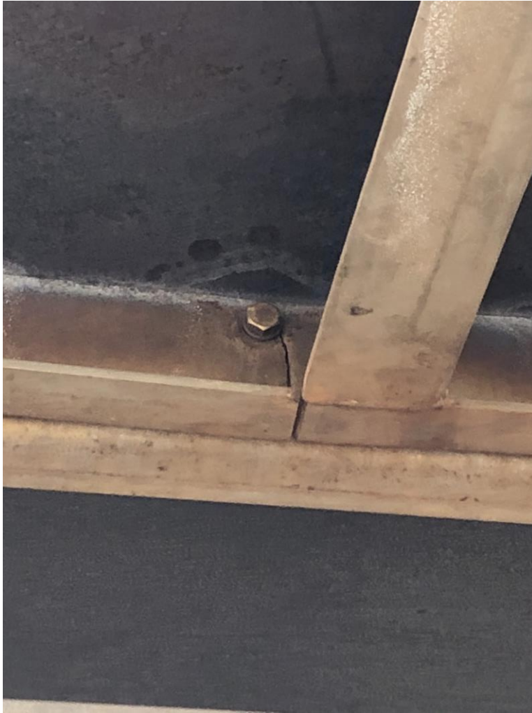
Figure 4: Cracking of exhaust structural support member, CS5 U2 (August 2019)
