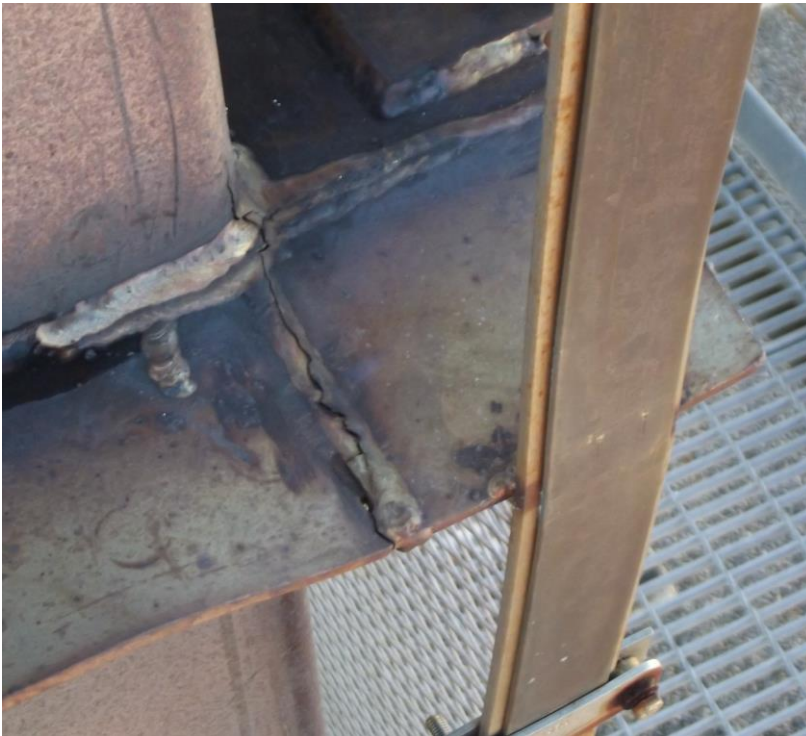
Figure 6: Sectional flange cracking CS8 Unit 1 (2020)
