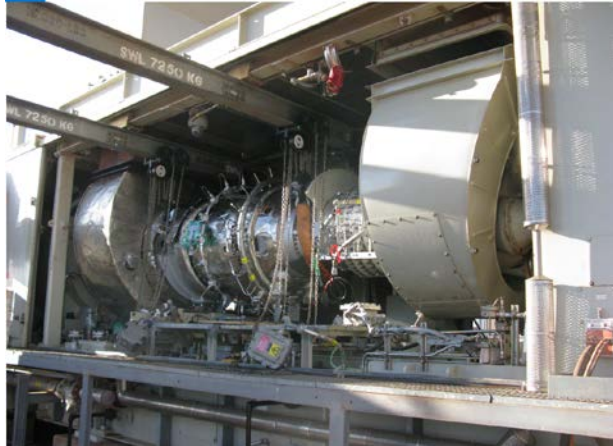
Figure 1.2: Gas turbine replacement
