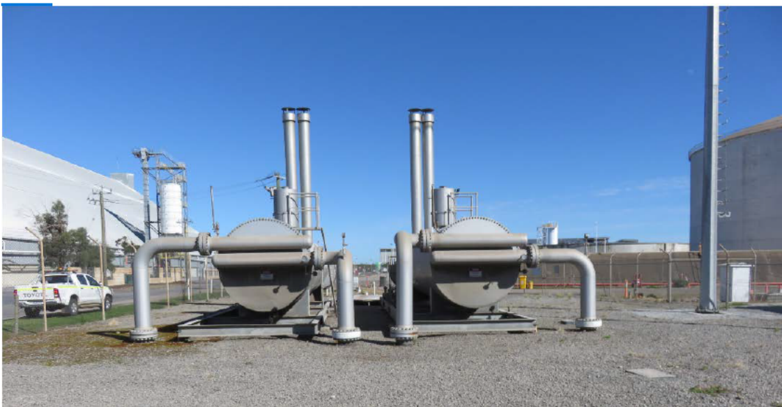
Figure 1.1: Kwinana Power Station Heaters to be decommissioned
