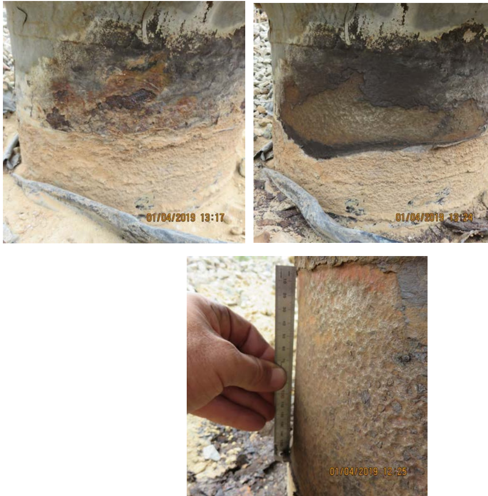
Figure 1.1: Photos of interface corrosion detected at facilities – features hidden behind the tape wraps
