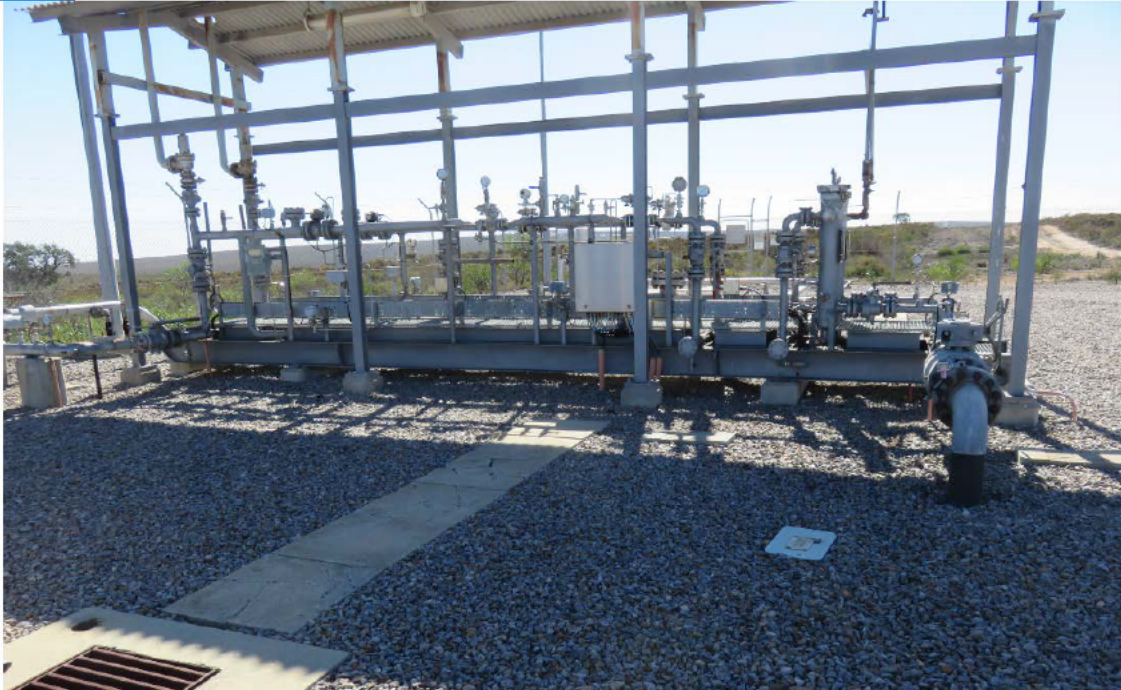
Figure 1.2: Eneabba meter station to be decommissioned
