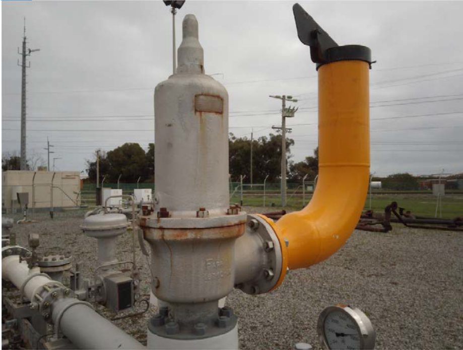
Figure 1.2: Pressure relief valve
