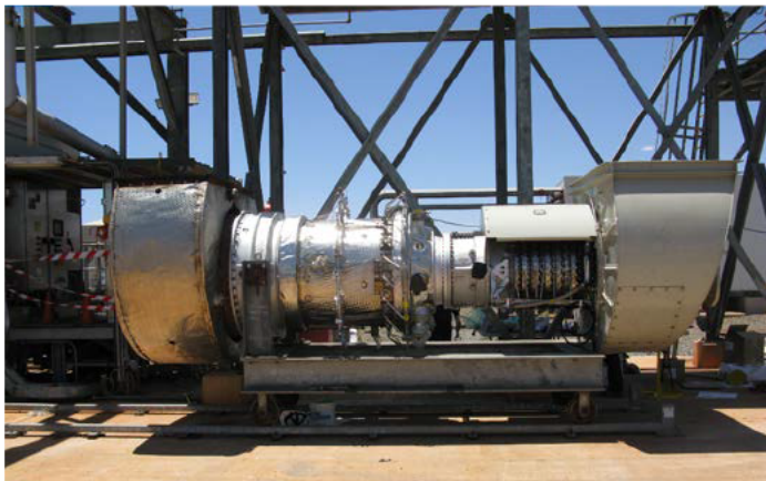
Figure 1.1: Gas turbine removal
