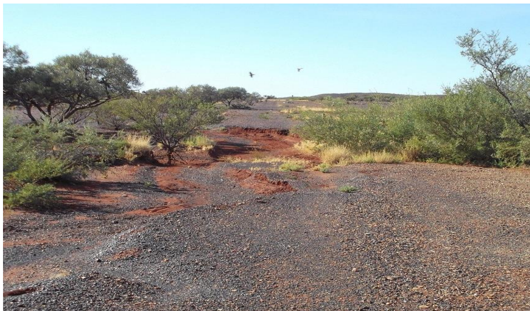
Figure 1: Scouring damage to the vehicle access at GGP Kilometre Point 247
