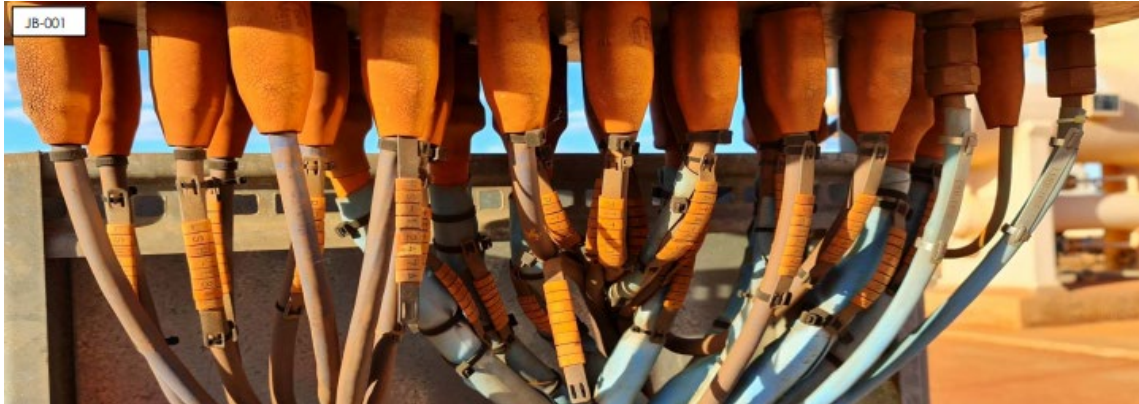
Figure 4.7.3 Example of defect at Paraburdoo Compressor Station. 24 cables without labels.
