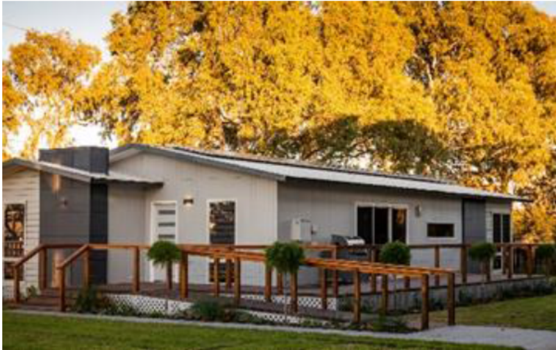
Figure 5: Hybrid Home at the ATCO Jandakot facility
